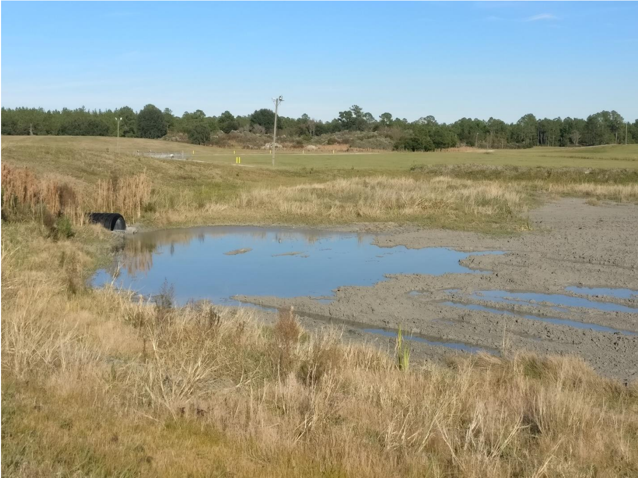
Figure 10. Ponding of Contact Water in the Northern Edge of the Cell 4 Basin Area
