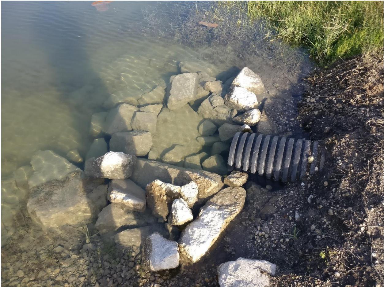
Figure 6. CCR in Northern Drainage Ditch
