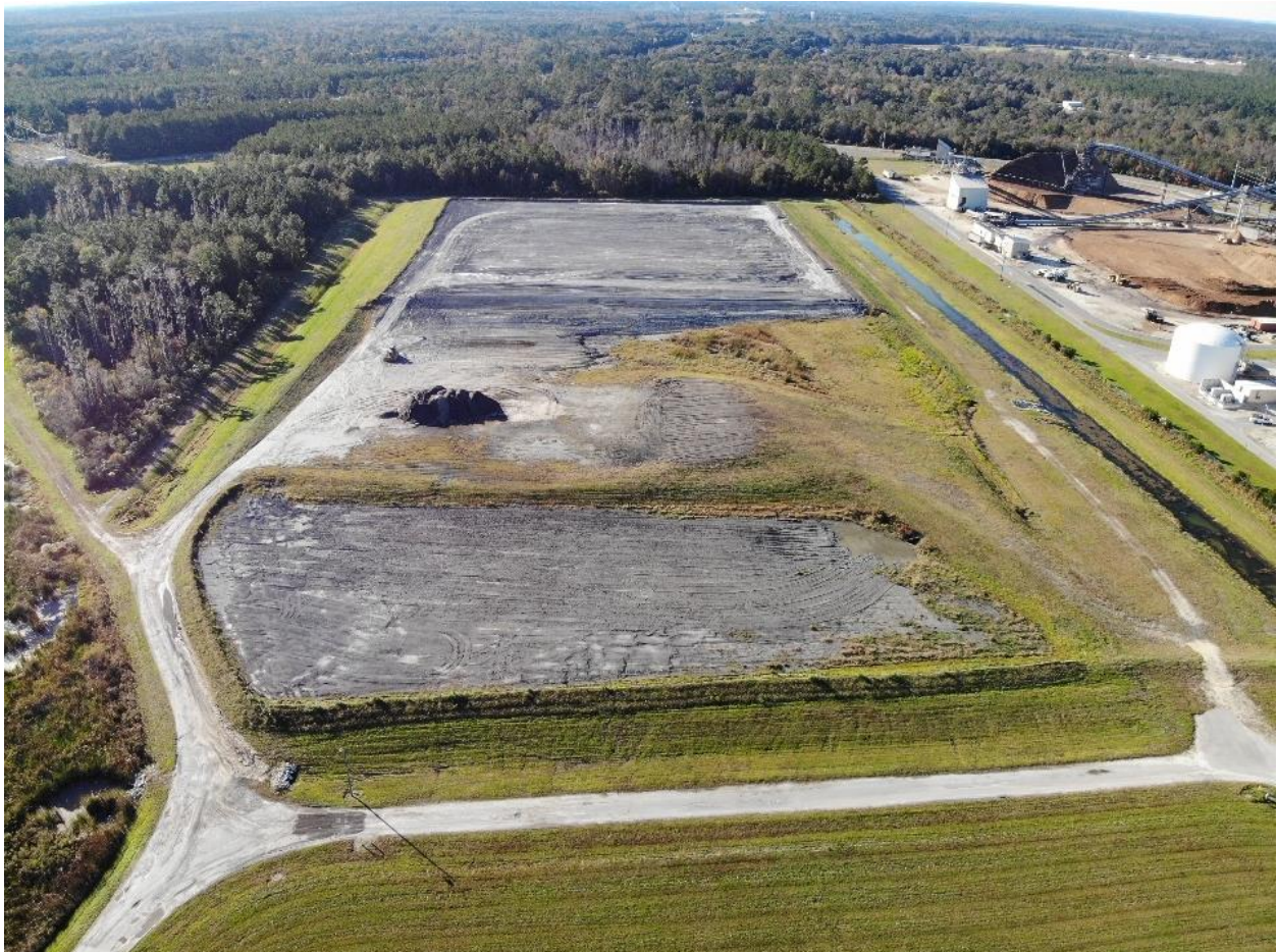
Figure 2. Aerial Image of CCR Landfill Facing West (IWCS 2018b)
