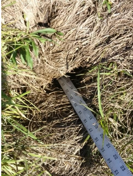
Figure 5. Forage Holes and Depths Observed on External Slopes of the Surface Impoundment System and Pump Back Ponds
