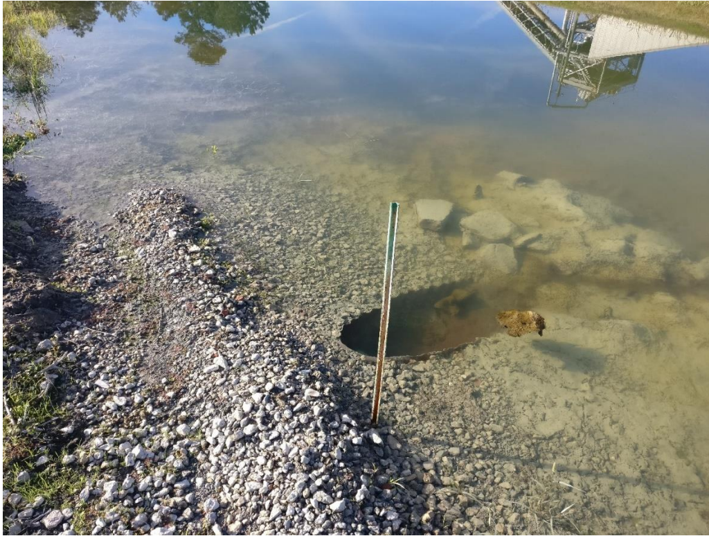
Figure 9. An Inundated Underdrain
